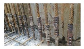
between reinforcing bars. Different sizes of reinforcing bars can be spliced with this system. This mechanical splice can also be used for joining reinforcing bars to structural steel components. Portable and bench type cold swaging press machines are provided by Regbar Construction. Typical applications include splicing tunnel eye bars, splicing of the column bars (or shearwalls), splicing of the beam bars, future extensions and segmental pours of concrete, repair applications.
