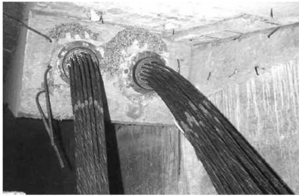
Fig. 4.1.1—Typical seven-wire prestressing strand (courtesy of HDR Engineering).
