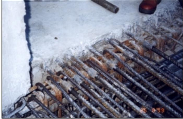
(b) Splicing of all slab main top bars
