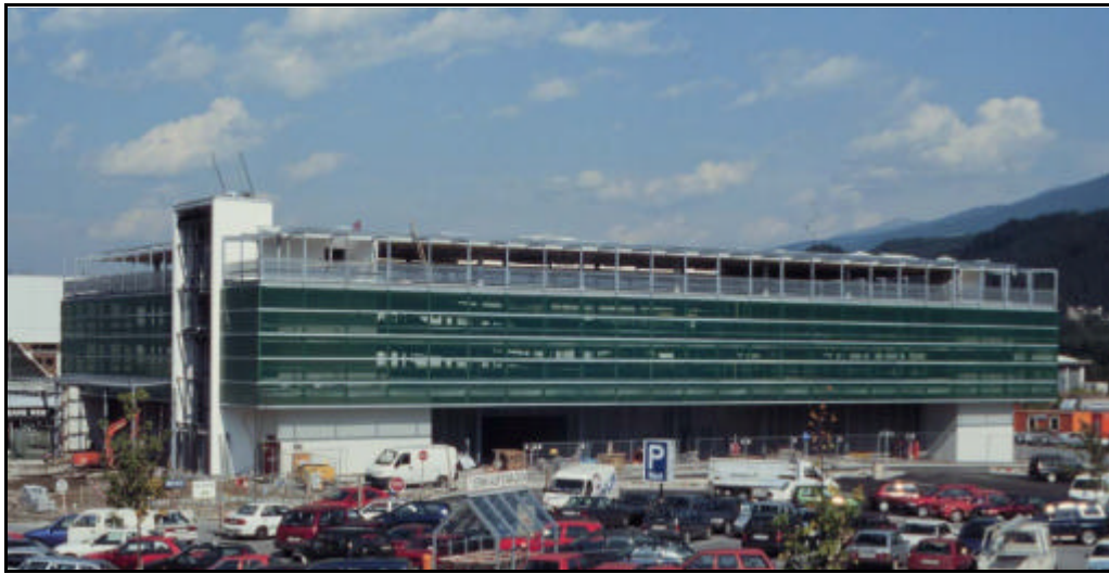
Figure 26 General view of the parking deck [8]
