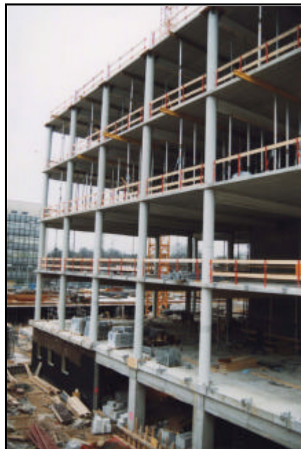
Figure 3 Columns and slabs on site (Citibank Duisburg, Germany) [8]
