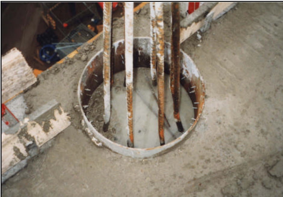
Figure 13 Tubular column with shot fired nails as shear connectors and reinforcement on site (Citibank Duisburg, Germany) [8]
