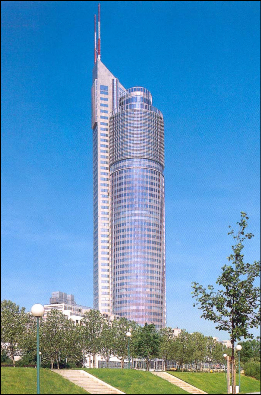
Figure 23 Millennium Tower Vienna (Austria) [8]
