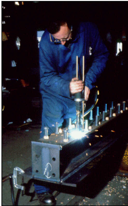
Figure 11 Welding of the shear connectors (headed studs) [9]
