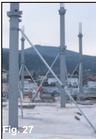
Figure 27 Erection of composite columns over 2 storeys
