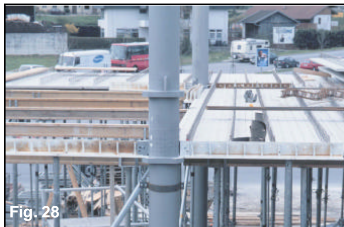
Figure 27 Erection of composite columns over 2 storeys
