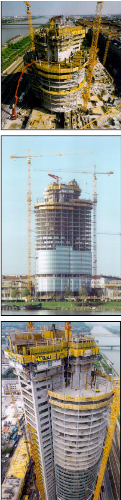
Figure 24 Construction progress (total erection time: 8 months) [8]
