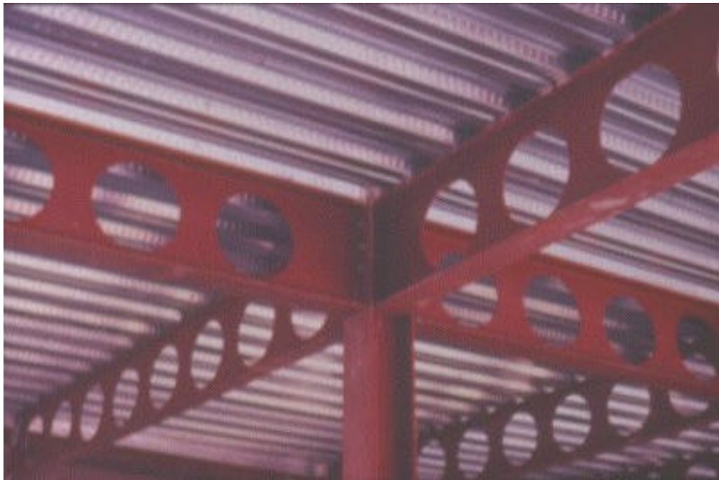
Figure 6 Cellular and castellated beams
